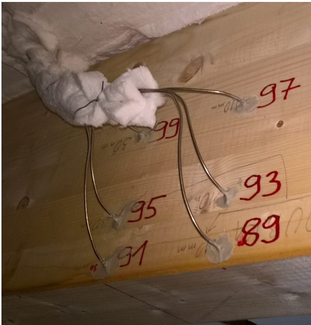
Fig. 13. Wiring to sensors.
